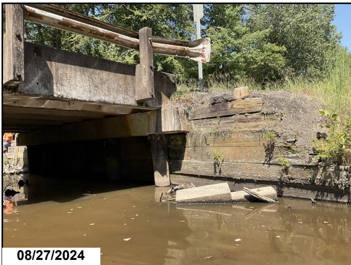
Bent 3, Right end, 1LF spall CS3, bridge rail end post has broken off the end of the cap.
