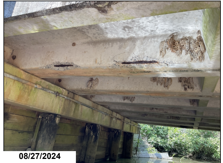
Span 1, Unit 7 Left leg, 1' back of mid span, 2LF exposed rebar CS3. 2' ahead of Bent 1, 2LF exposed rebar CS3.
