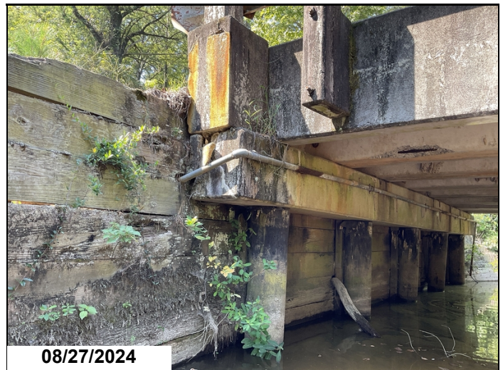
Bent 1 Right end, 1LF spall CS3
