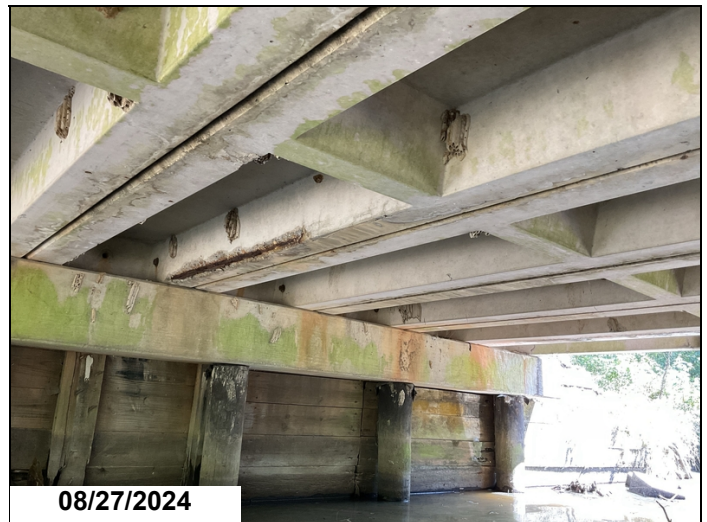
Span 2, Unit 3, Right leg, ahead of mid span 3LF cracking CS3. Back of Bent 3, 5LF exposed rebar CS3.
