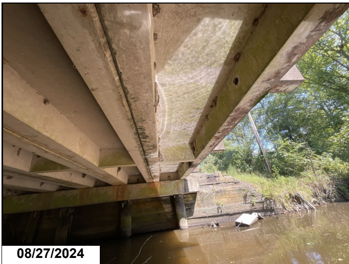
Span 2, Unit 7 Left leg, ahead of Bent 2, 9LF cracking CS3. 2LF spall CS2.
