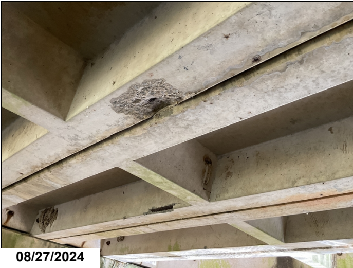
Span 1, Unit 4, Right leg, 1' back of mid span, 1LF spall CS3.
