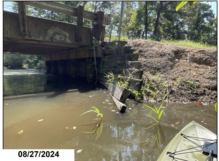
Bent 1, 10' of the left end, scour of embankment behind the backwall causing timbers to be bowed ahead in to the channel. 10LF scour CS3.
