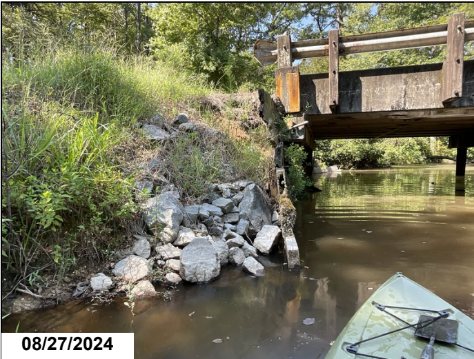
Bent 1, 10' of the right end, scour of embankment behind the backwall causing timbers to be bowed ahead in to the channel. 10LF scour CS3.
